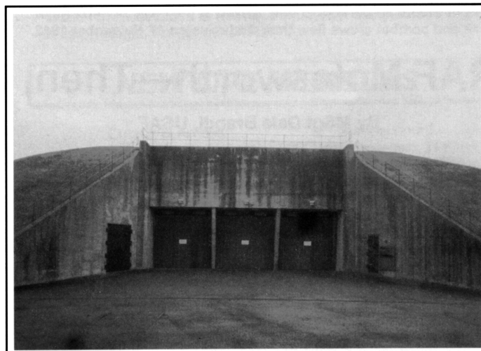
THE GROUND LAUNCH CRUISE MISSILES of the 303rd TMW were stored in bunkers capable of withstanding the shock of a near direct hit in a nuclear attack. The empty bunkers are still in place.
